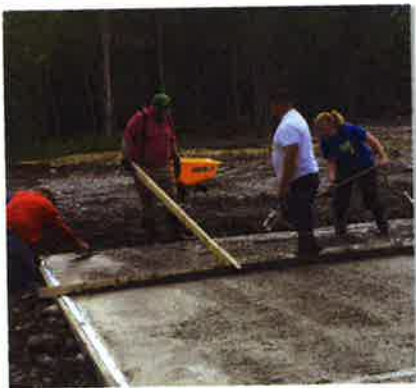
WORKING ON THE SLAB
