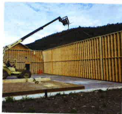
WALLS PUT IN PLACE!
